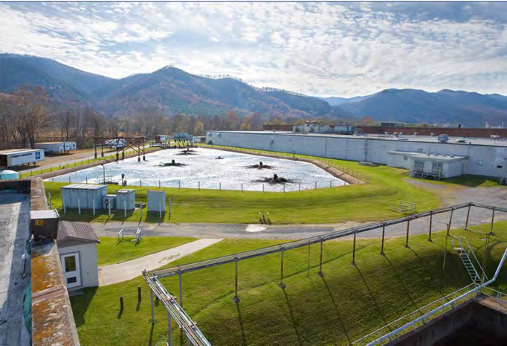
Our carpet tile manufacturing plant in Glasgow, Virginia.
